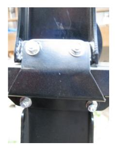
On the bottom of the antenna post use 2 @ 5/16" x 3/4" with washers and locking nuts.
